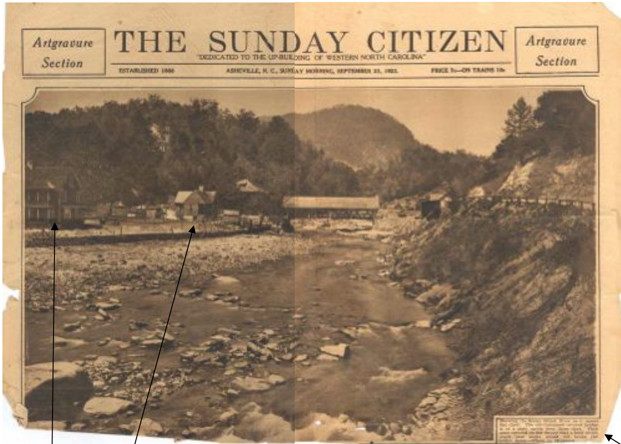
NEWSPAPER CLIPPING FROM 1923: “Showing the Rocky Broad River as it passes Bat Cave. The old-fashioned covered bridge is of a style rarely seen these days. They were covered on the theory that a load which could pass under would not break the bridge down”—photo by Higgason. This bridge was built after the 1916 Flood.
